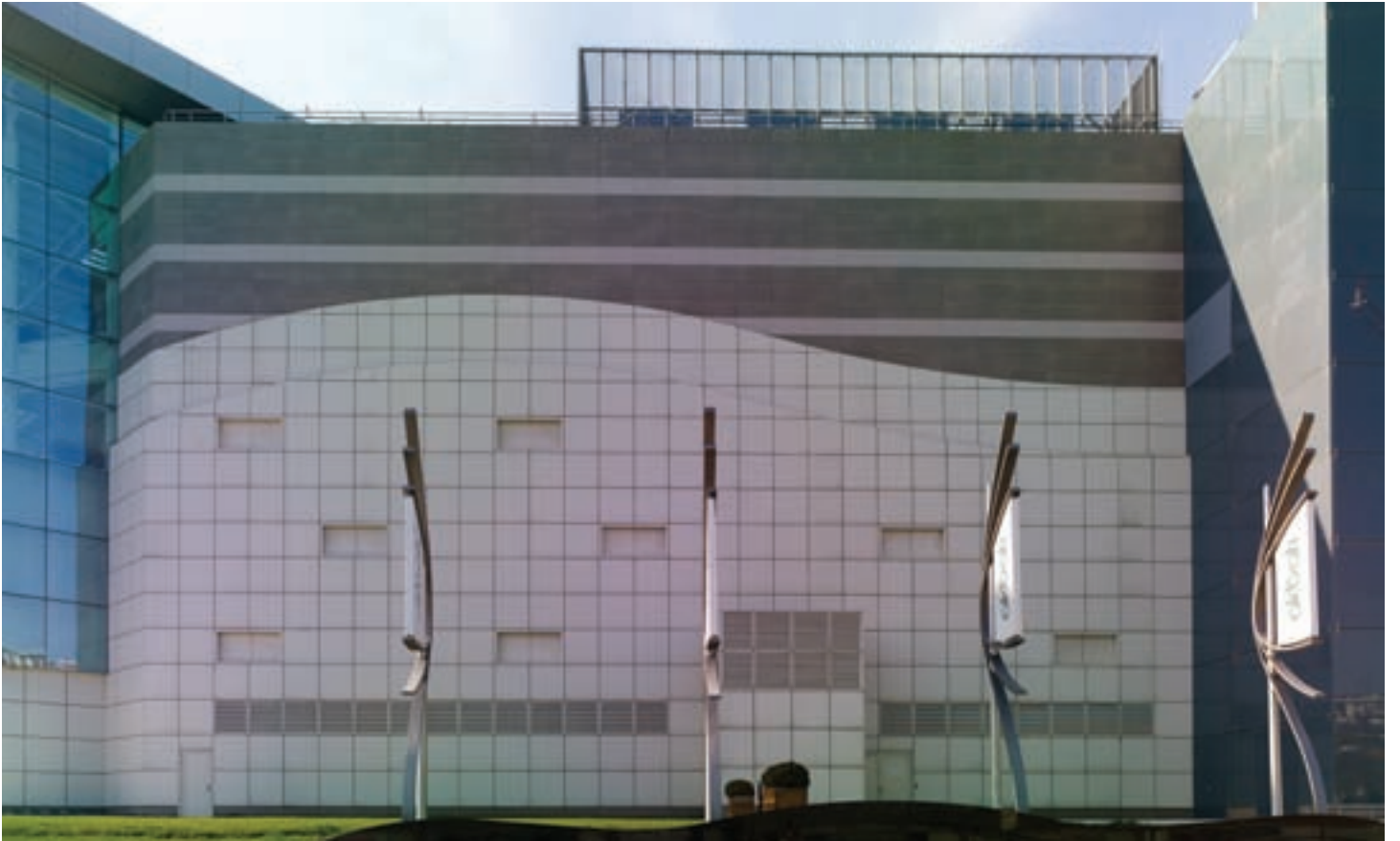
Akbatı AVM, Esenyurt / İstanbul — 60x120cm Heraklia Stone Beyaz - 60x120cm Apollon Stone Yeşil / Klipsli Sistem Akbatı AVM, Esenyurt / İstanbul — 24"x48" Heraklia Stone White - 24"x48" Apollon Stone Green / Clips System Mimar : Seçkin Mimarlık — Architect : Seçkin Architectural Office
