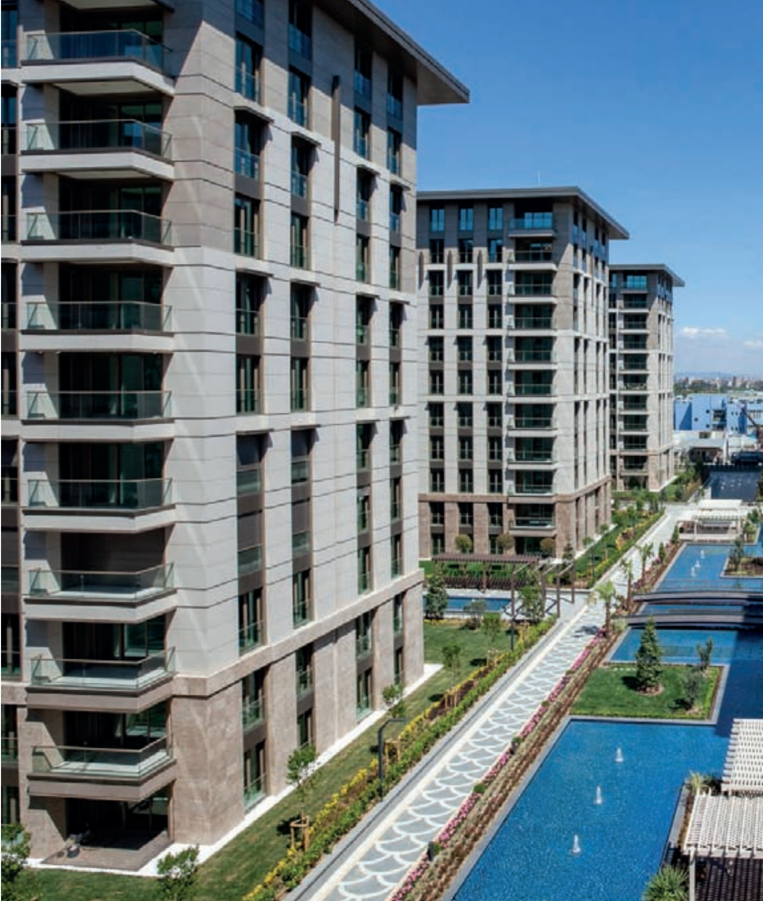
Avrupa Konutları Topkapı / İstanbul — Kalesinterflex 3mm fit limestone, 3mm fit sandstone gy305 / Gizli Klipsli Sistem Avrupa Residences Topkapı / İstanbul — Kalesinterflex 3mm fit limestone, 3mm fit sandstone gy305 / Hidden Clips Fitted Facade System Mimarlık: Viva Mimarlık — Architect : Viva Architects
